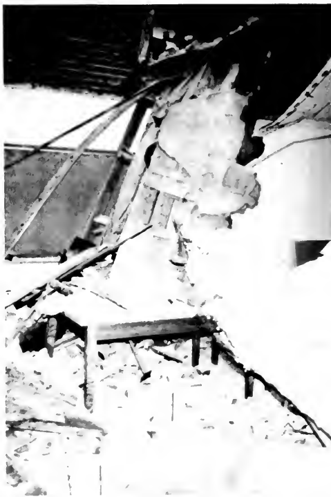
Photo 2. Los Angeles High School. Portion of brick parapet fell through roof into adjacent classroom wing.
